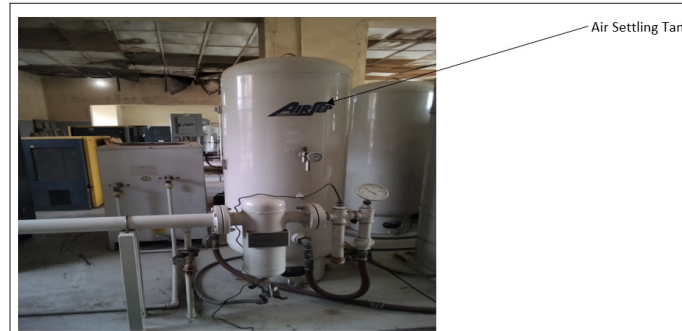
Figure 2: Air Settling tank (MAWP 200psi at 150F, MIWP -20 F at 200psi)
