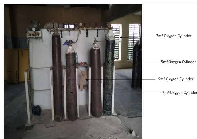
Figure 5: Cylinder Filling Ramp
