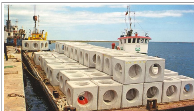
Figure 1: Reef Transport to the Installation Zone, by Mota-Engil 2025
