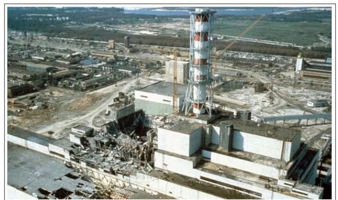
Figure 1: Partial Destruction of Chernobyl Power Plant
