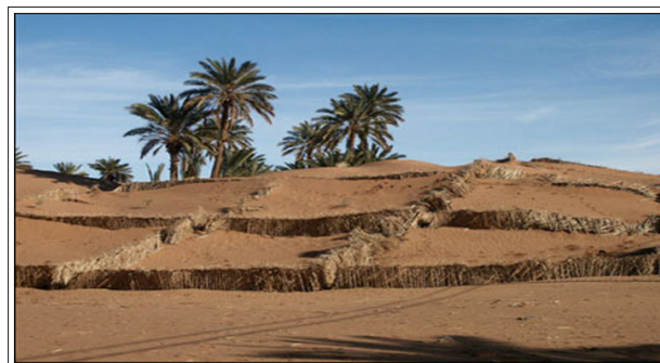
Figure 9: Methods for Mechanically Sustaining Sand Utilizing Palm Frond Squares
