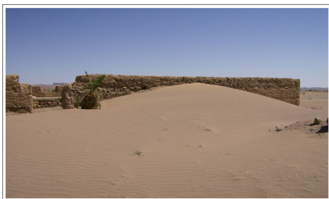
Figure 6: Demonstrates Methods of Mechanically Stabilizing Sand by Using Walls to Shield Farmland Against Sand Intrusion
