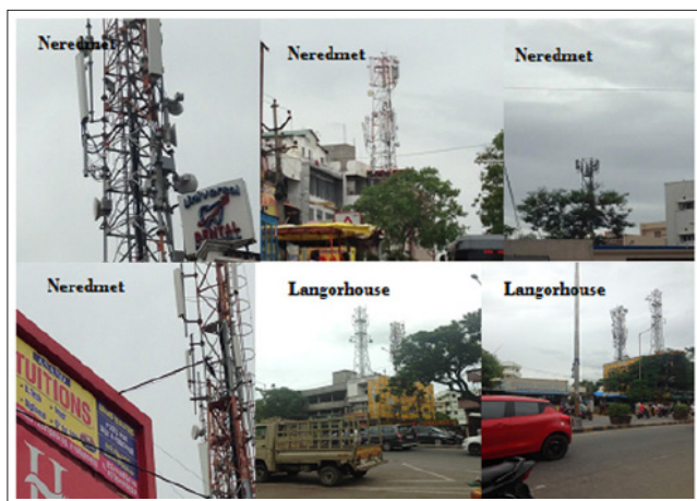
Figure 5: Mobile towers very close to residential / commercial areas in Hyderabad (India).
