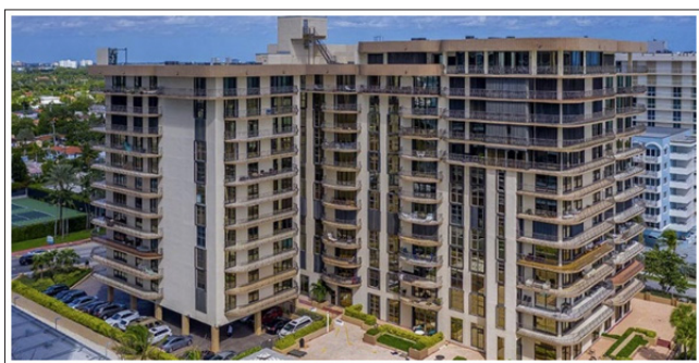
Image 1: is the photo of the Florida building before it collapsed.
