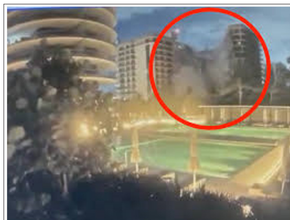
Image 2: Photo of the Florida building during the incident. [13]
