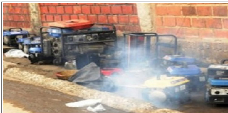
A Typical Source of Power Supply in the Nigerian Market
